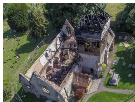
The burnt out shell
